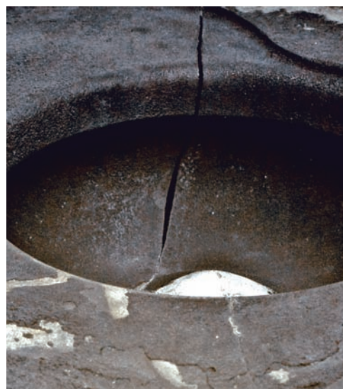
Fig. 1 Cracks in the bowl rim
